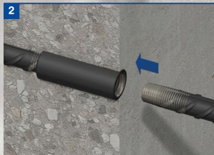
2 After casting the concrete and when ready to extend, remove the plastic end cap from the coupler. Position the continuation bar in the sleeve and rotate the bar into the coupler.
