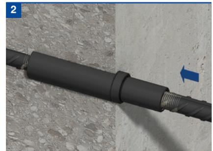
Position the continuation bar as near as possible to the coupler fitted to the cast-in bar.
